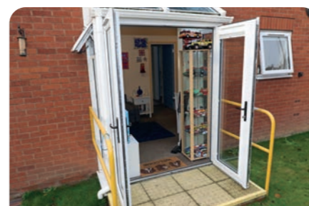
Image: The small patio entrance to a flat at Hammond Court.
